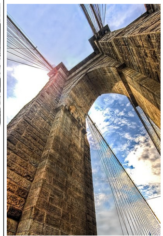
Figure 4: Towers of the Present Day Brooklyn Bridge, 2008
