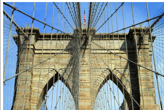
Figure 6: View of suspender cables of the bridge, 2013
